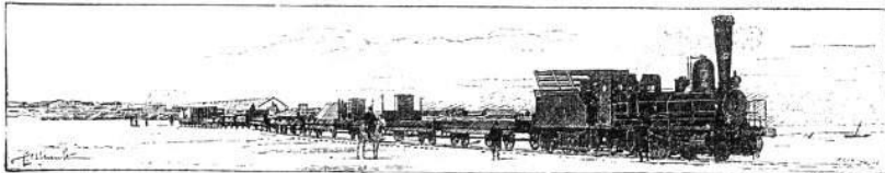
A RAILWAY ON THE ICE—PROVISIONAL CONSTRUCTION TRAIN CROSSING THE FROZEN IRTISCH RIVER.
